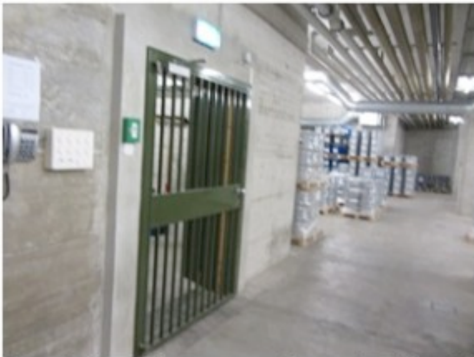
Deeply buried storage vault, north of Zurich. Lots of heavy steel and thick concrete.
